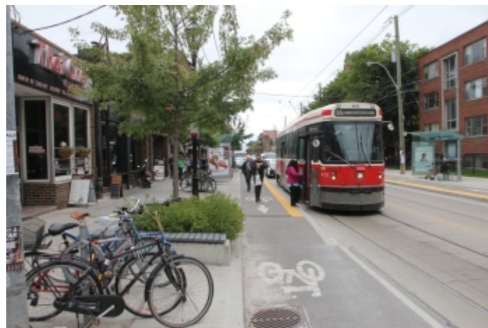
Figure 4. Illustration of a bus boarder-type configuration at a tram stop, Toronto, Canada 3 .
